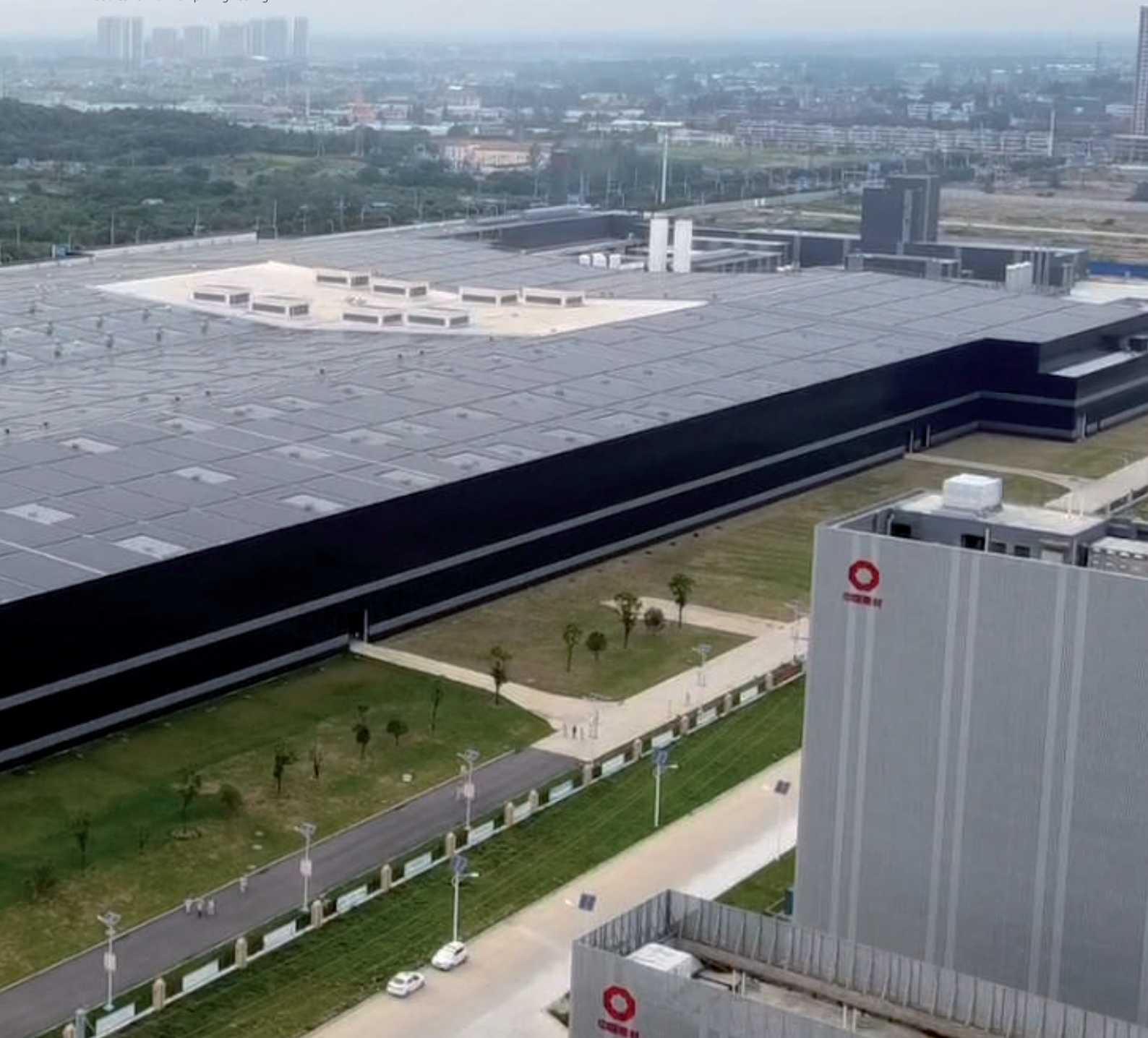
Figure 4.1. World's largest integrated thin-film solar cell building demonstration project in Anhui, China. Source: China Triumph Engineering.
