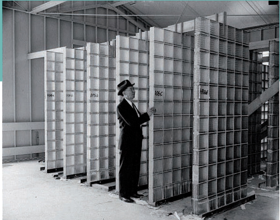
Figure 6.4. Bureau of Standards making extensive tests of glass building blocks (Washington DC). Source: Library of Congress.
